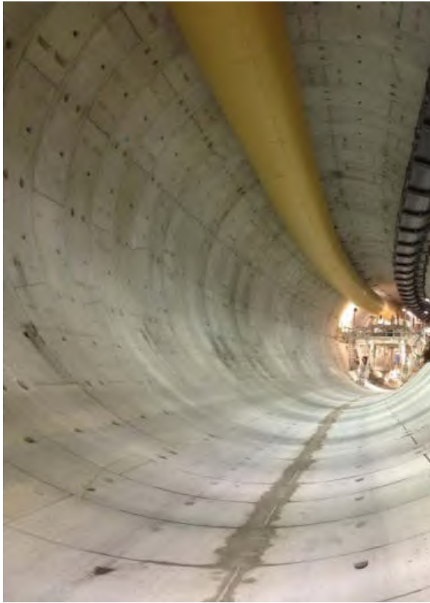
Figure 4.20 A – Example of precast tunnel liner segments.
