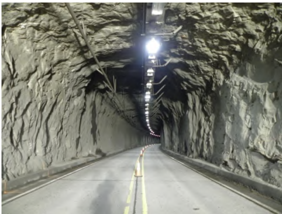
Figure 4.27 – Various unlined rock tunnels.
