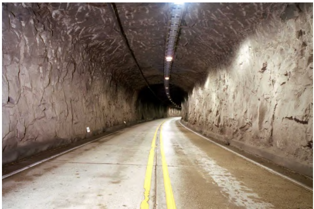
Figure 4.27 – Various unlined rock tunnels.
