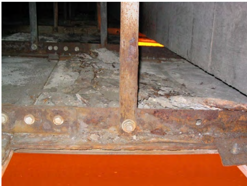
Figure 4.37 – Hangers and ceiling girders exhibiting moderate to heavy rust and minor section loss.
