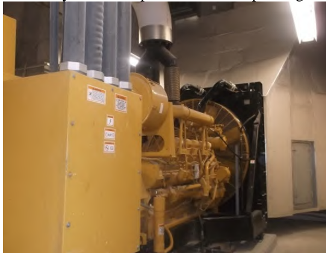
Figure 4.62 – Emergency Generator.
