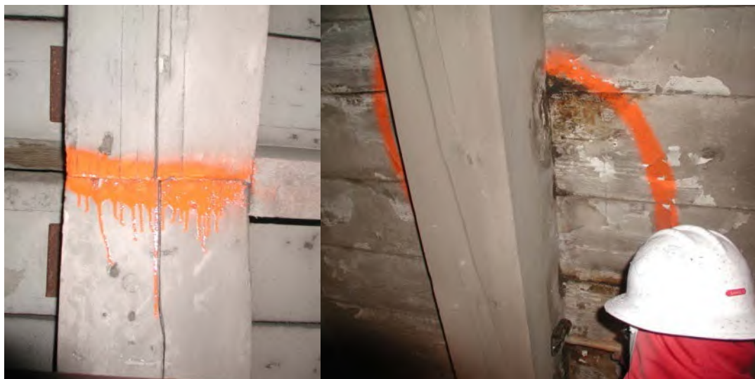
Figure 4.17 – Examples of defects in timber liners
