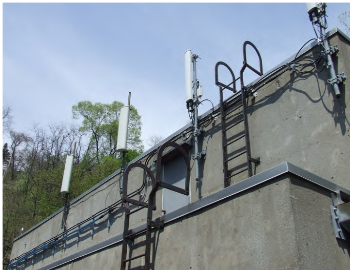
Figure 4.42 – Ancillary building: with metal ladders to roof.
