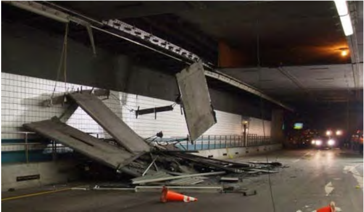
Figure 4.35 – Overhead items such as ceiling panels must be inspected to prevent fatalities.
