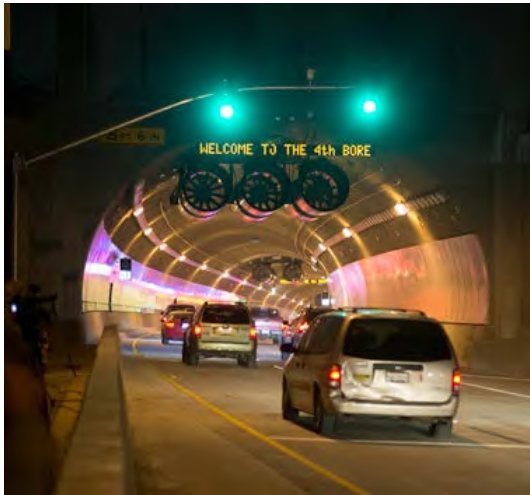
Figure 4.33 – View of tunnel with metal panel finish covering concrete liner.
