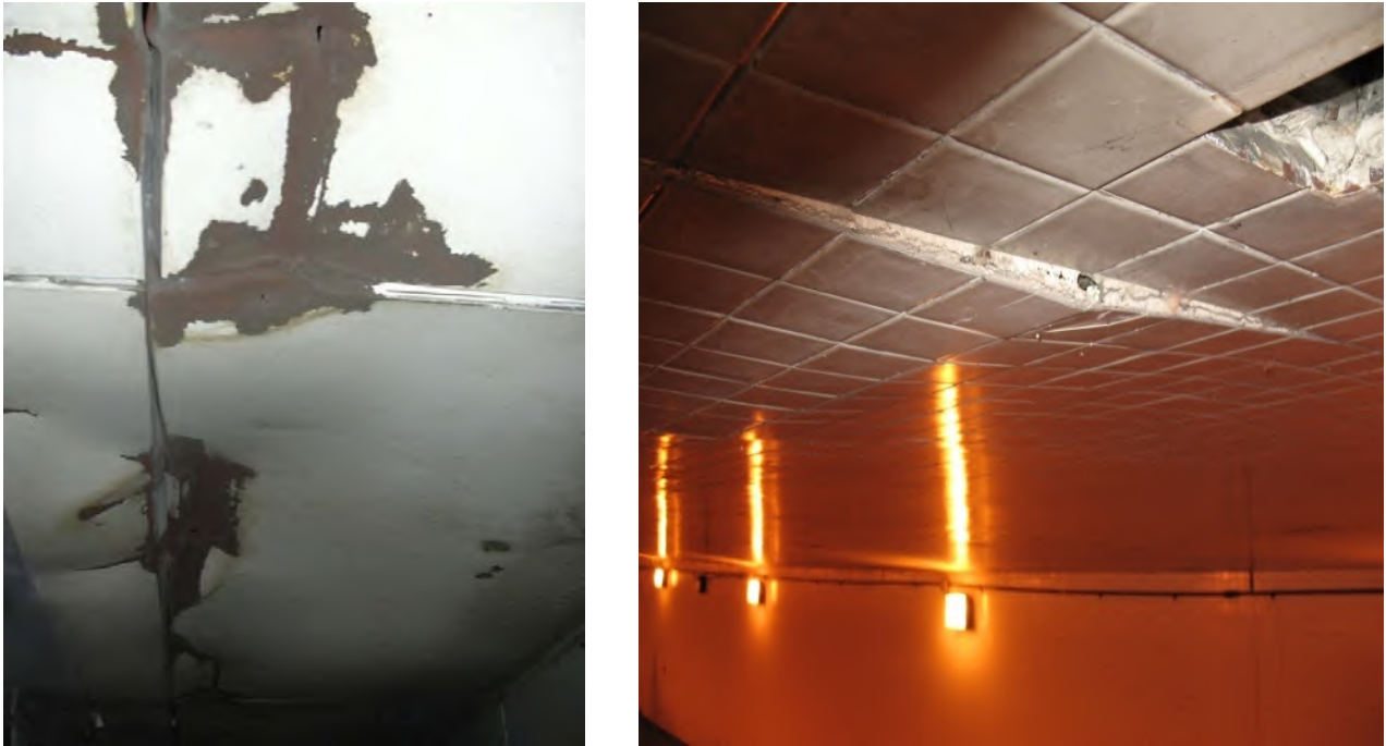
Figure 4.39 – Examples of damaged and deteriorated architectural finishes on underside of ceilings. Photo left is of damaged metal ceiling panels; right is deteriorated ceramic tile.
