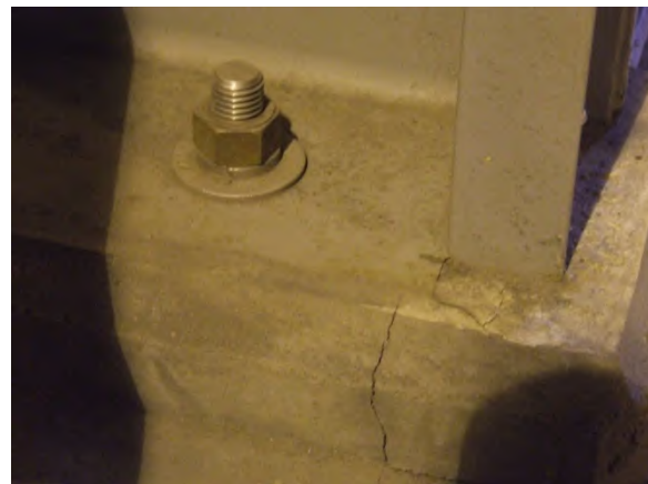
Figure 4.45 – Cracked machinery
