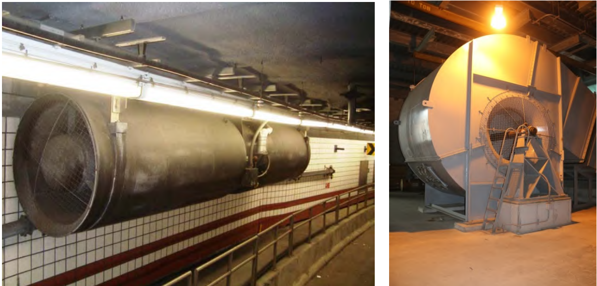
Figure 4.51 – Axial fan, left and centrifugal fan, right.
