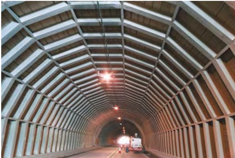
Figure 4.25 – New timber rib and lagging liner.
