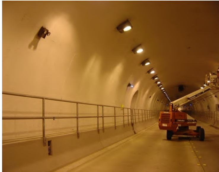
Figure 4.46 – Typical civil elements including wearing surface, traffic barrier, and pedestrian rail and walkway.
