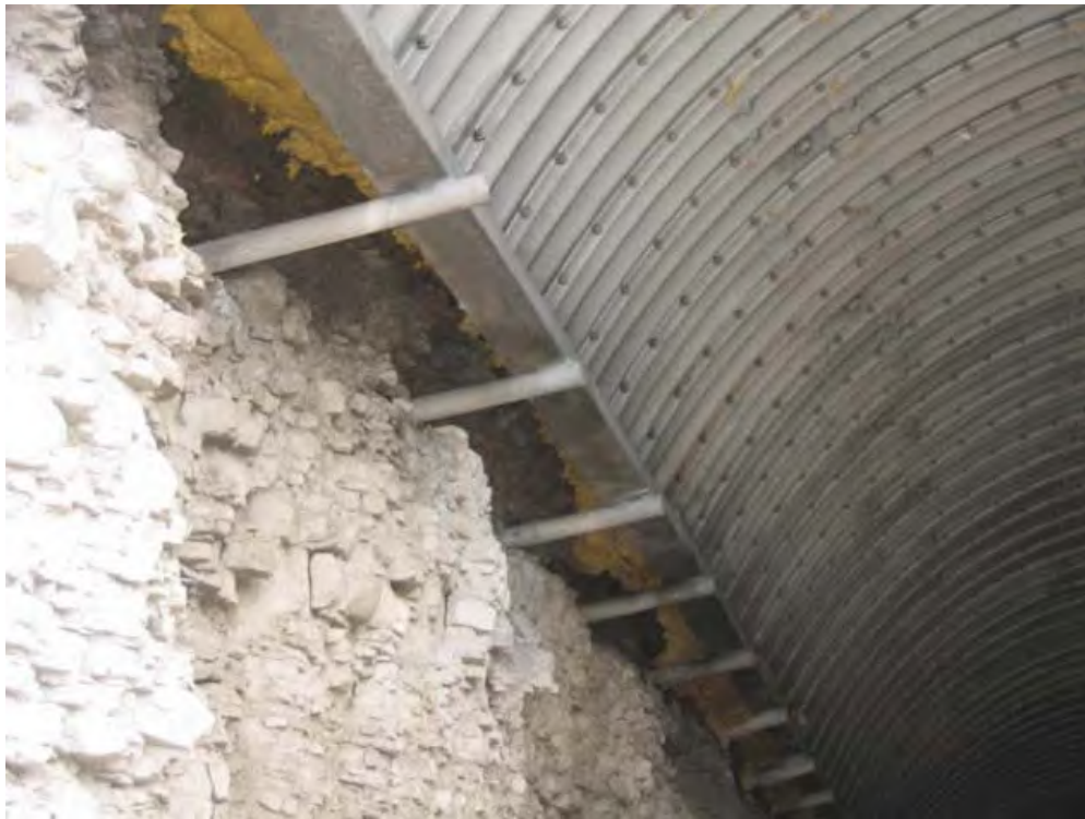
Figure 4.19 – Steel liner plate above the springline.
