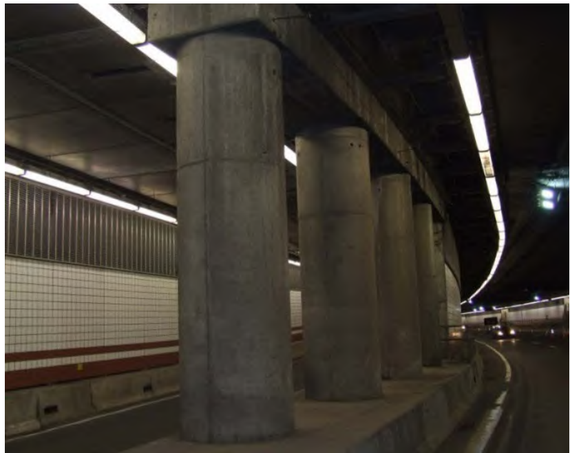
Figure 4.30 – Columns with bent cap.
