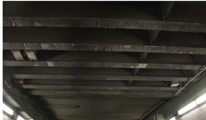
Figure 4.29 – Exposed roof girders.
