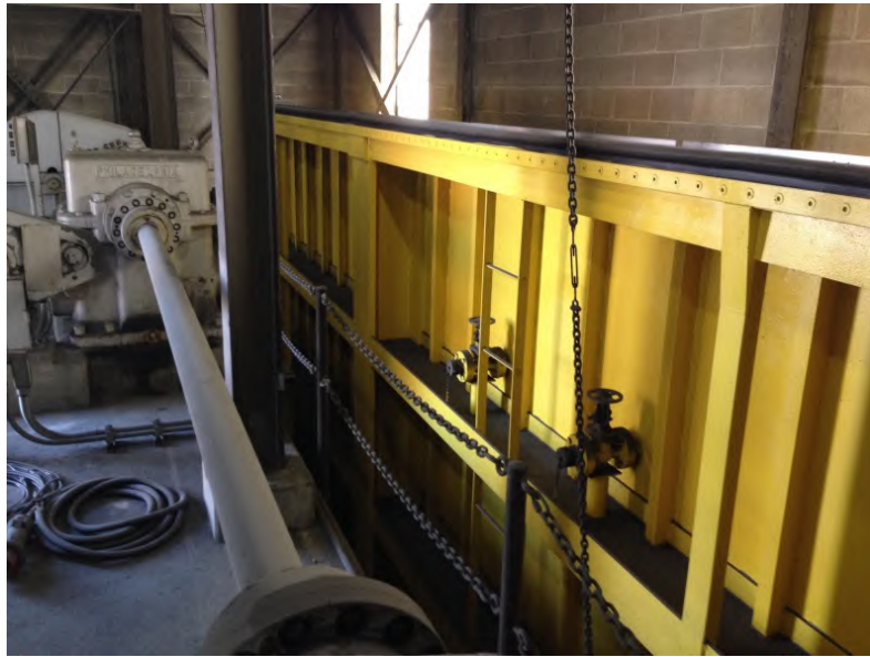
Figure 4.63 – Flood gate.
